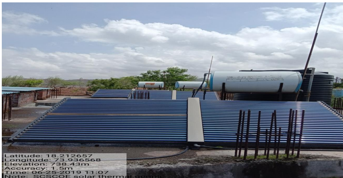
Photograph of Solar Thermal Water Heating System at Hostel block:
