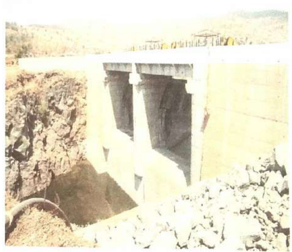
Photo No.6- Ogee spillway
