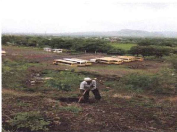
Non Teaching Staff During Digging.
