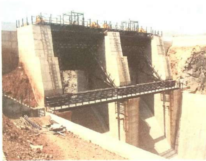
Photo No.6- Ogee spillway
