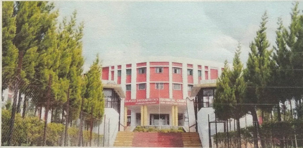
RDTC, SHRI CHHATRAPATI SHIVAJIRAJE COLLEGE OF ENGINEERING, DHANGAWADI, TAL: BHOR, DIST: PUNE (MAHARASHTRA)
