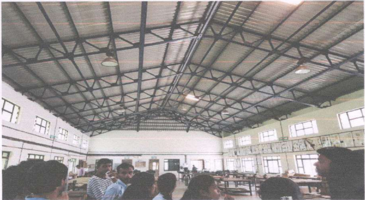
Photo No. 2- Sutar sir explain details of truss to student a
