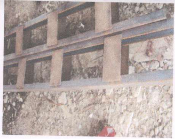
Photo No.3 -Column with battens
