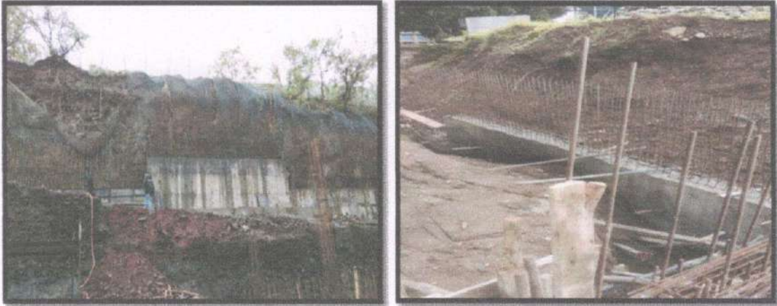
Photo No.1 Retaining Wall at construction site
