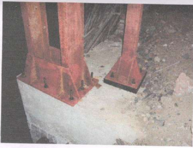
Photo No.2- Column base
