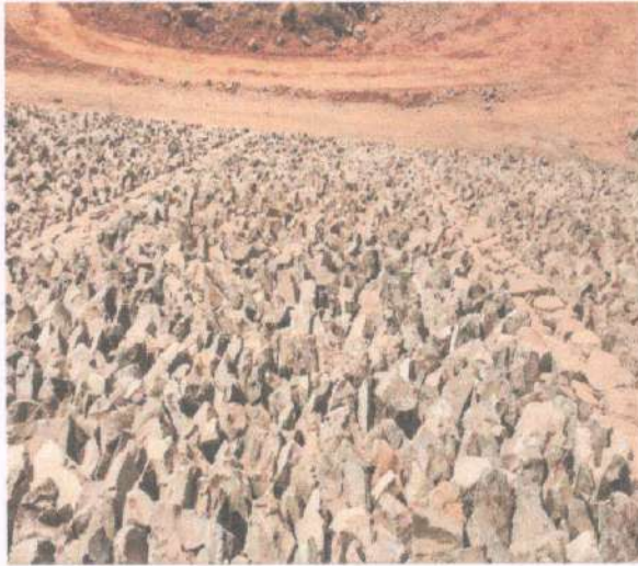
Photo No.4. -Needle and Flat pitching
