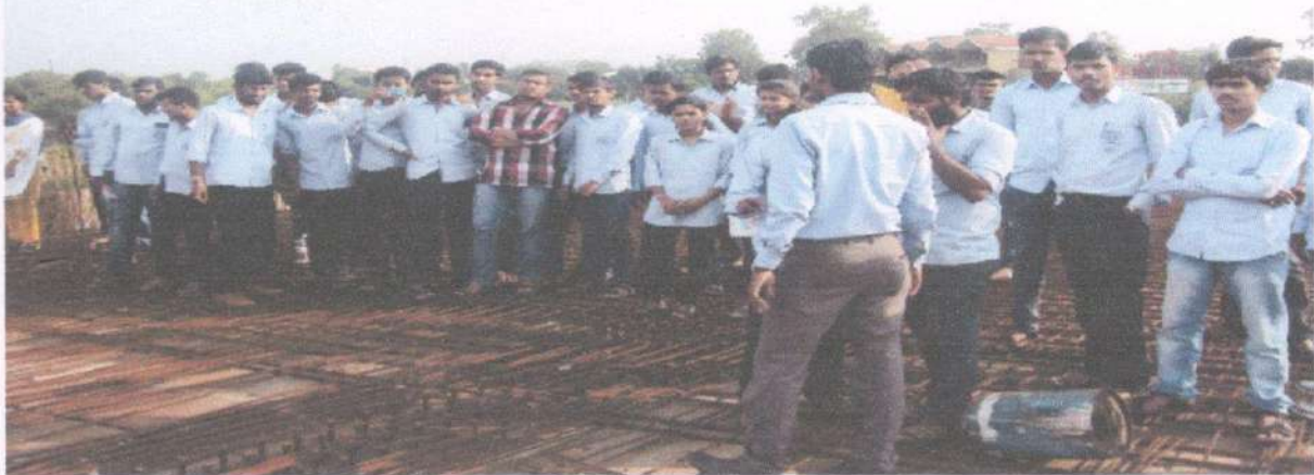
Photo No.2- Reinforcement detail
