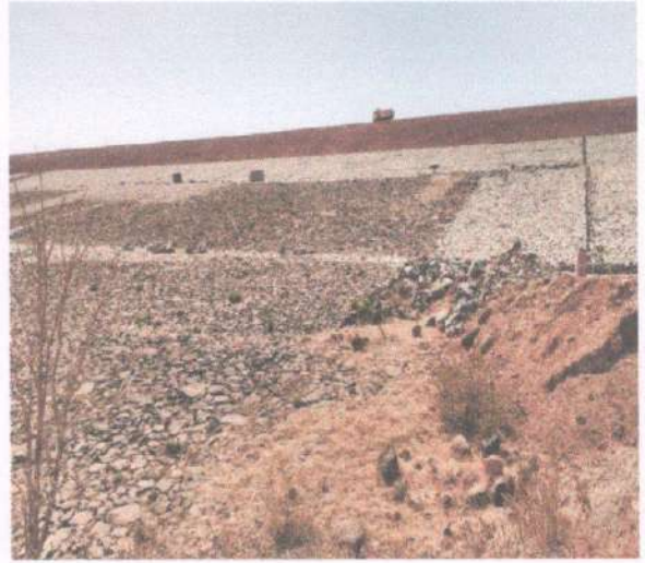
Photo No.4. -Needle and Flat pitching
