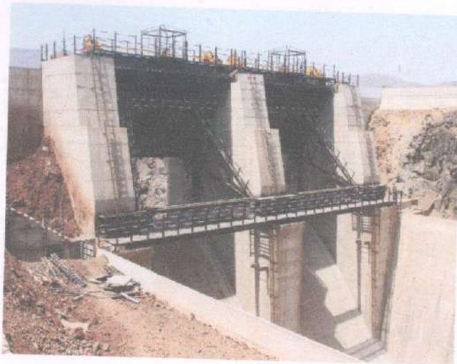
Photo No.6- Ogee spillway
