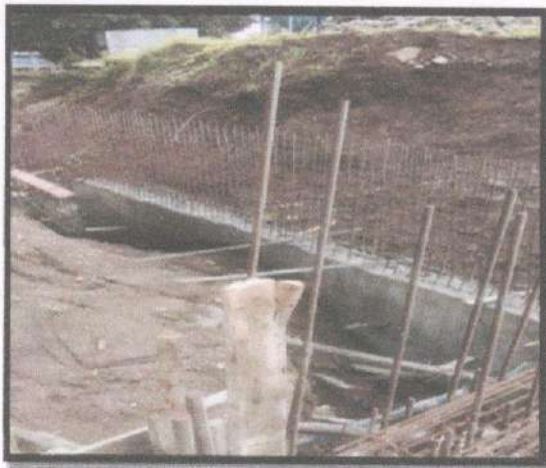
Photo No.1 Retaining Wall
