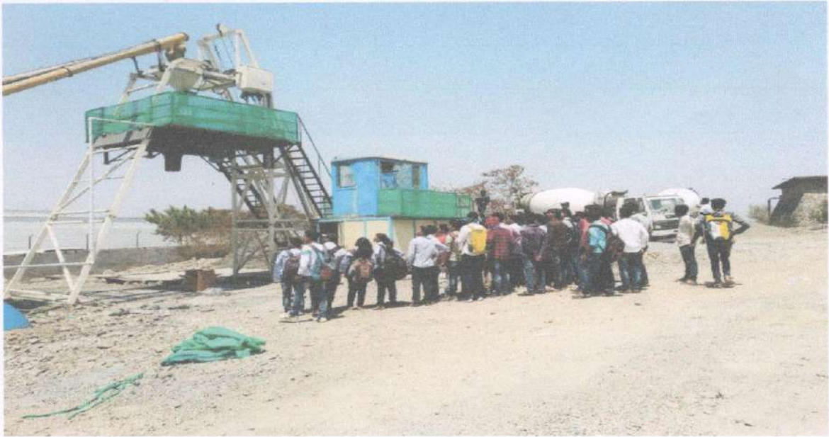
Photo No.1: Site Engineer explain process of RMC plant
