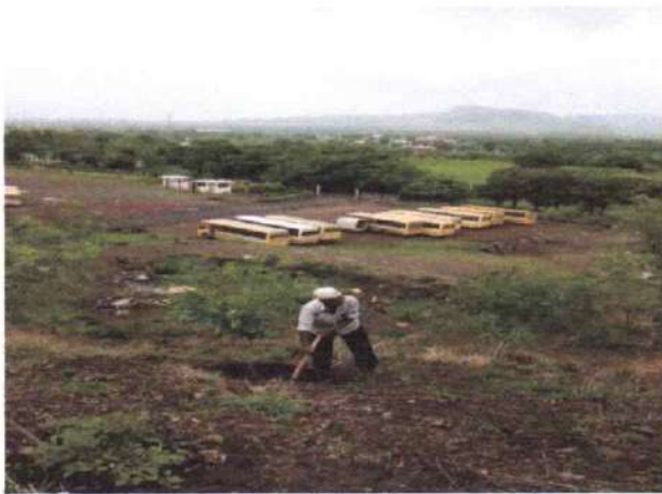
Non Teaching Staff During Digging.
