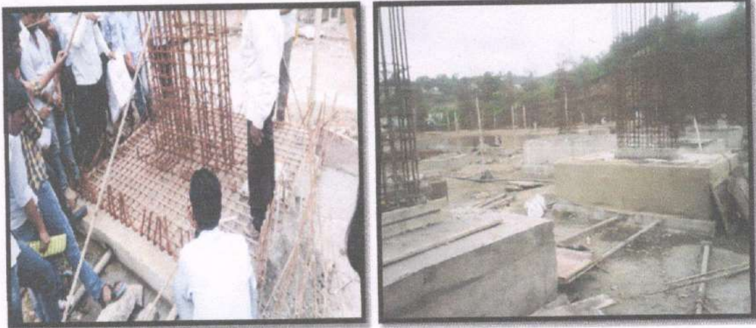
Photo No.1: Reinforcement and casting of combined footing
