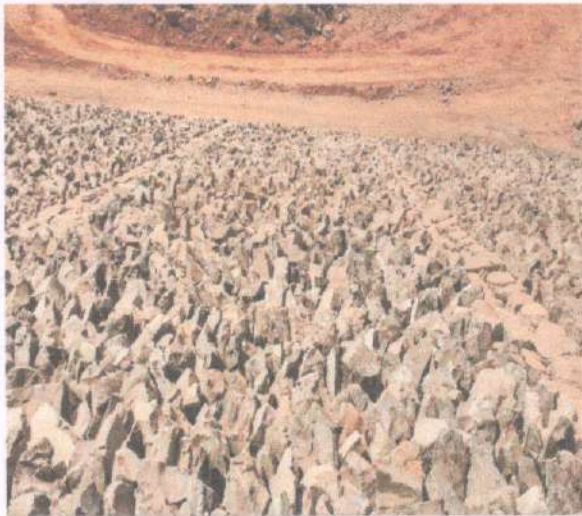
Photo No.4. -Needle and Flat pitching
