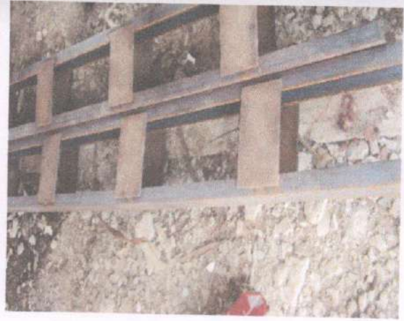
Photo No.3 -Column with battens
