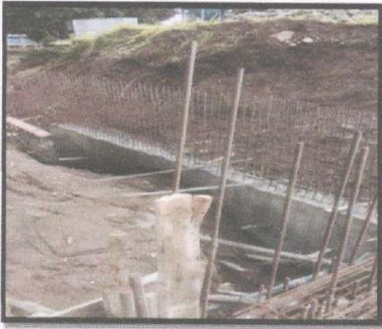
Photo No.1 Retaining Wall
