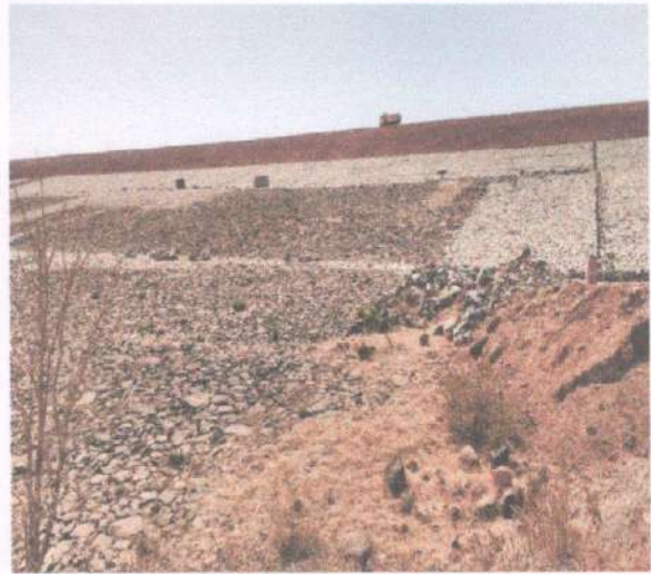
Photo No.4. -Needle and Flat pitching
