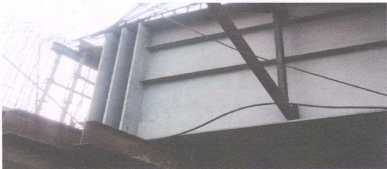
Photo No.3- Bearing and horizontal stiffeners
