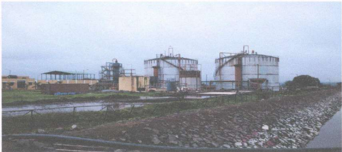
Photo No.2 -Photo at ETP Plant, Bhunj
