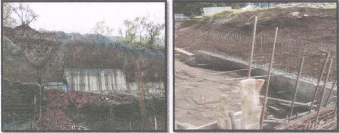
Photo No.1 Retaining Wall at construction site
