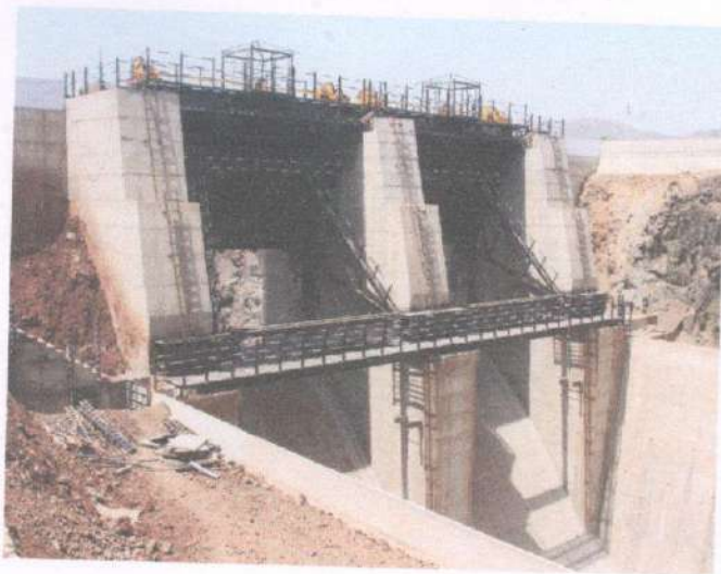
Photo No.6- Ogee spillway
