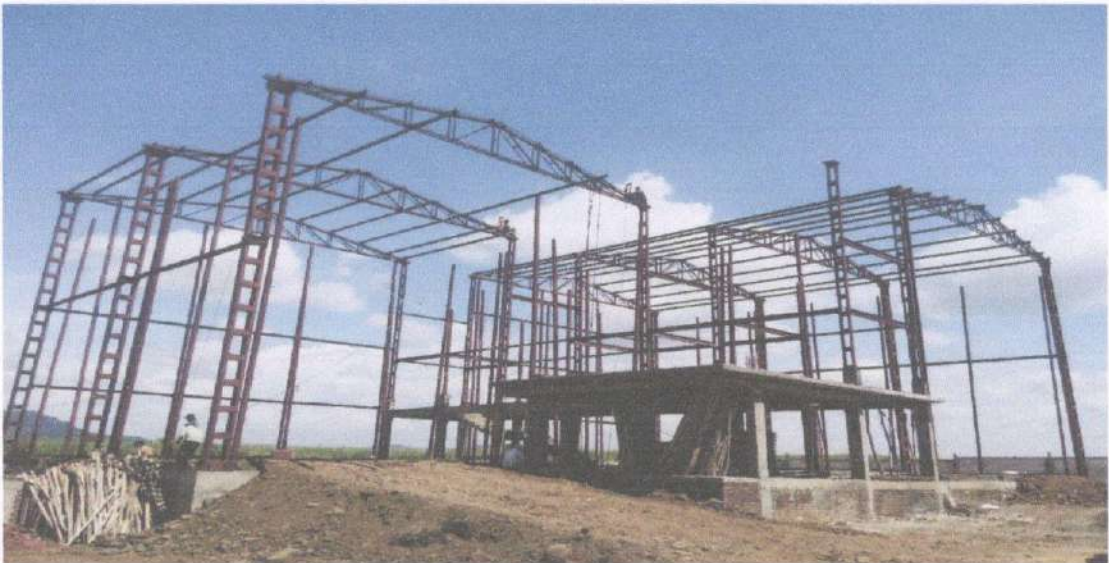
Photo No.1 -Sarsawati cold storage site
