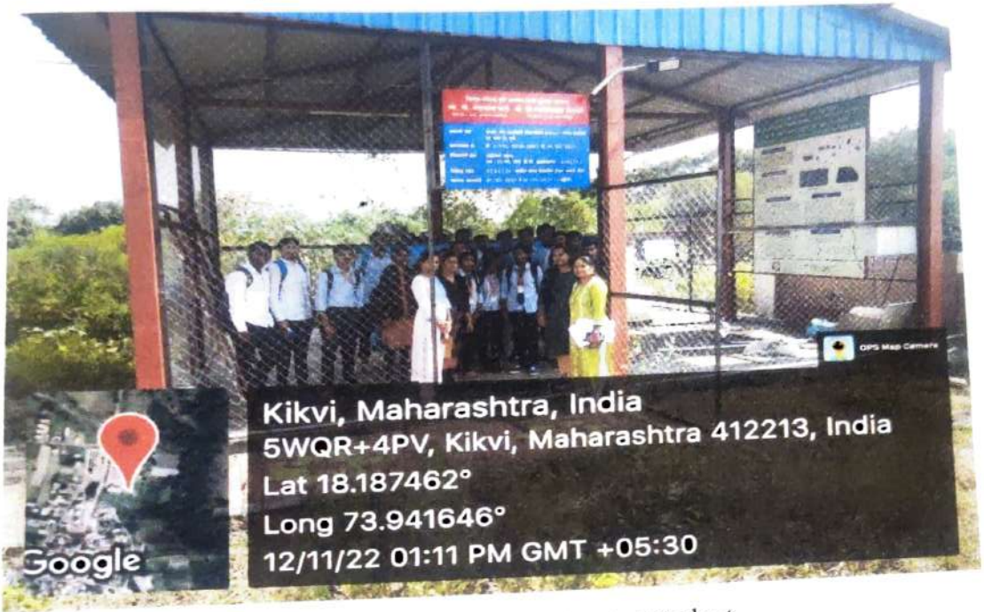
Fig.1: Package water treatment plant
