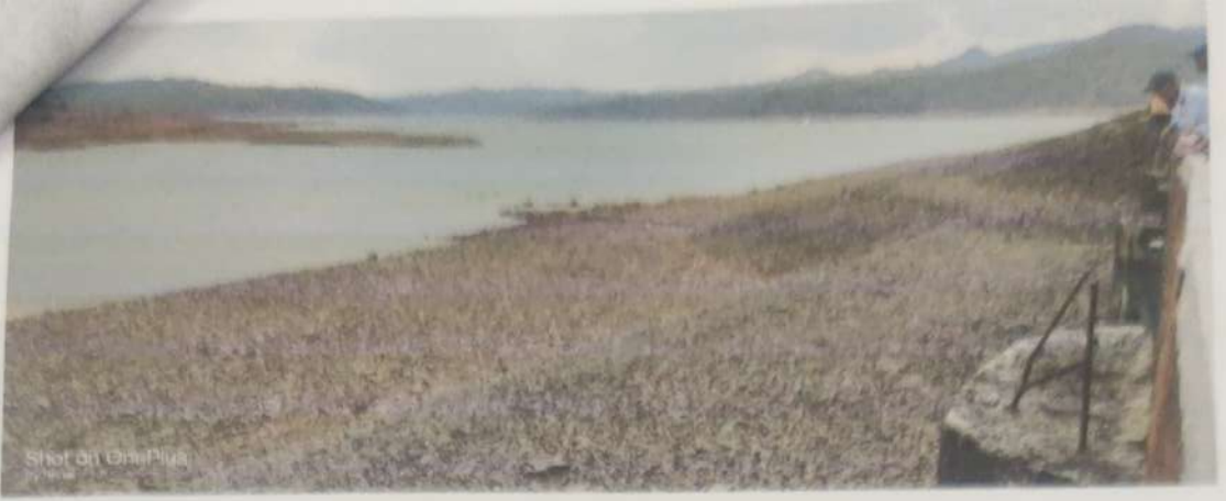
Photo No.3 . Needle and Flat pitching
