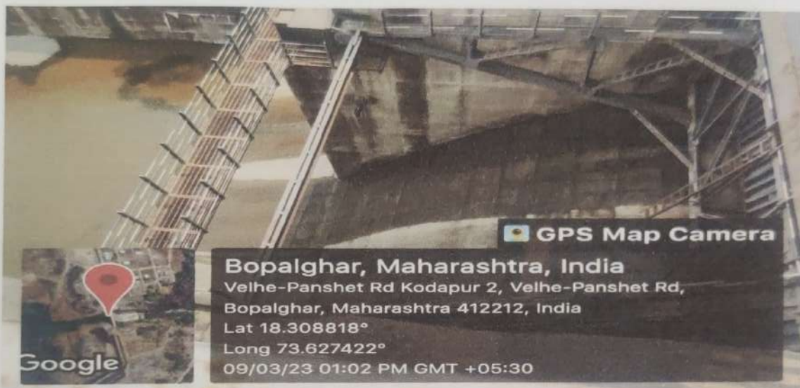
Photo No.2 . Ogee Spillway
