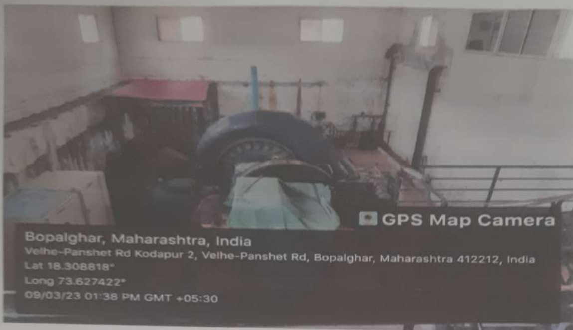
Photo No.1- Pelton Turbine
