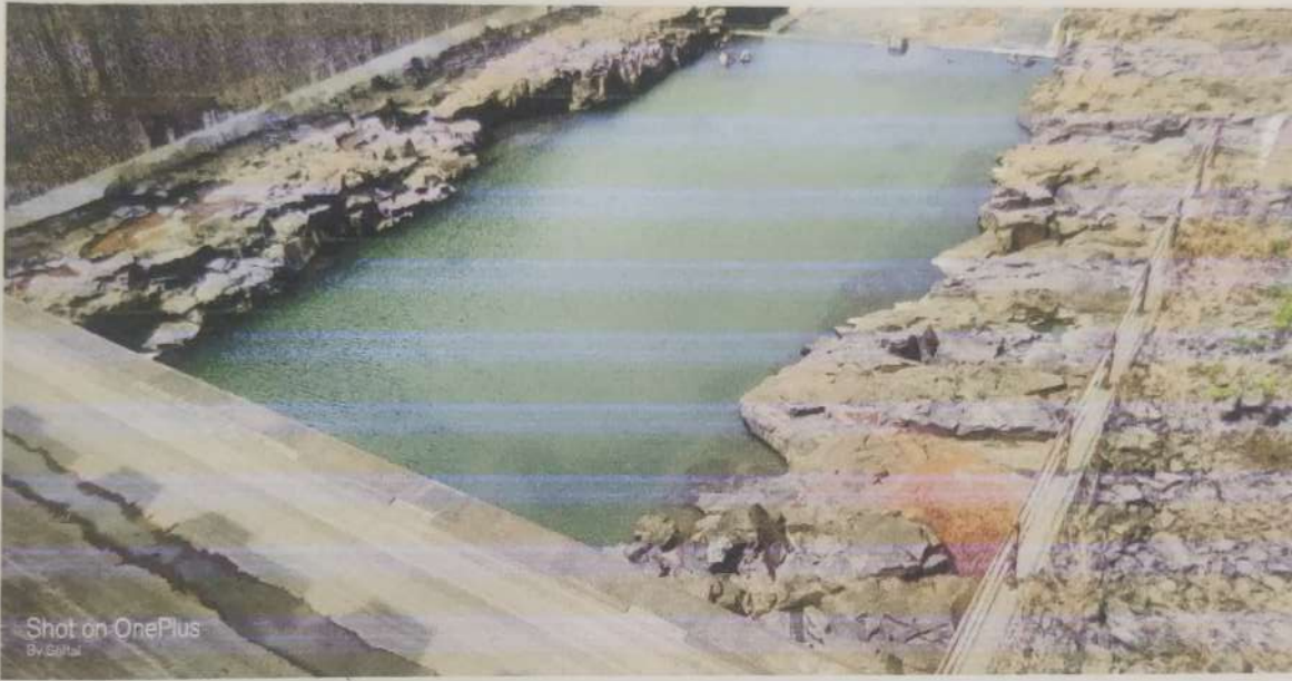
Photo.No.1-Stilling basin & Ogee Spillway
