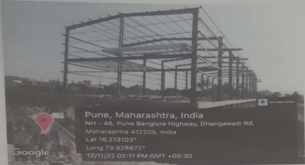
Photo No.1- Industrial Shed
