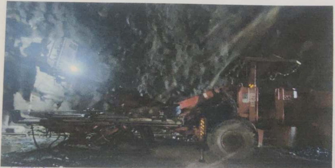
Photo : Tunnel Construction Equipment
