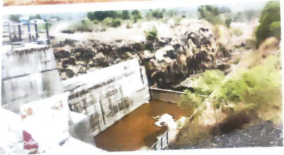
Photo :Ogee Spillway at Gunjawani dam
