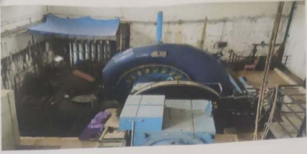
Photo No.1- Pelton Turbine
