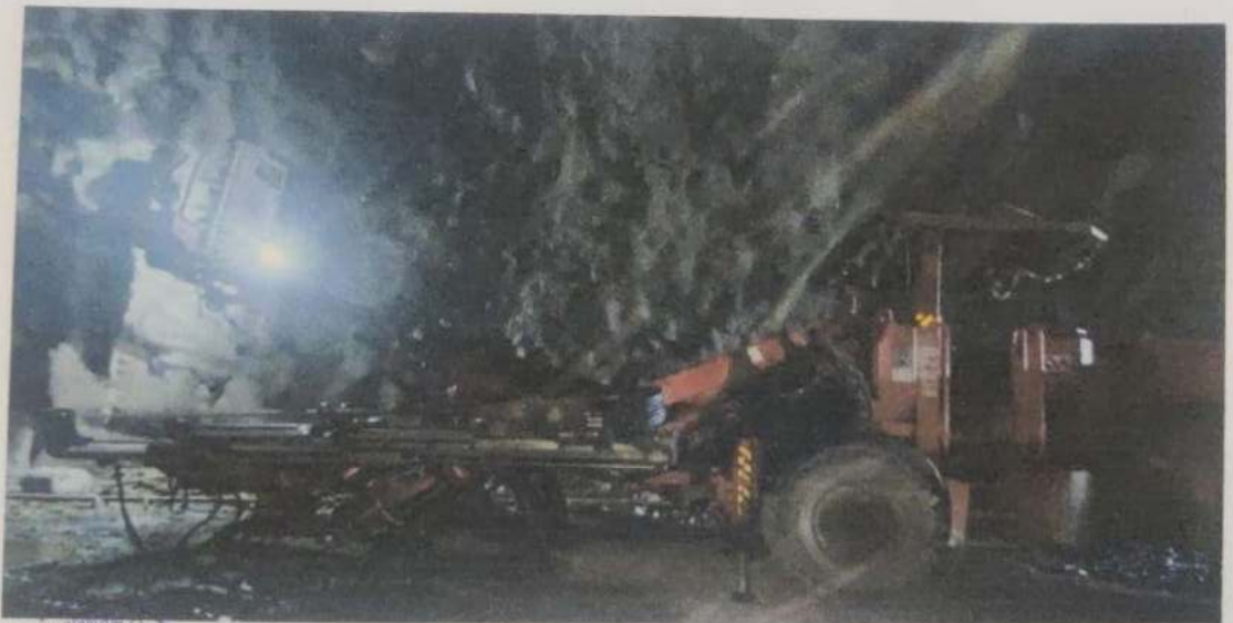
Photo : Tunnel Construction Equipment
