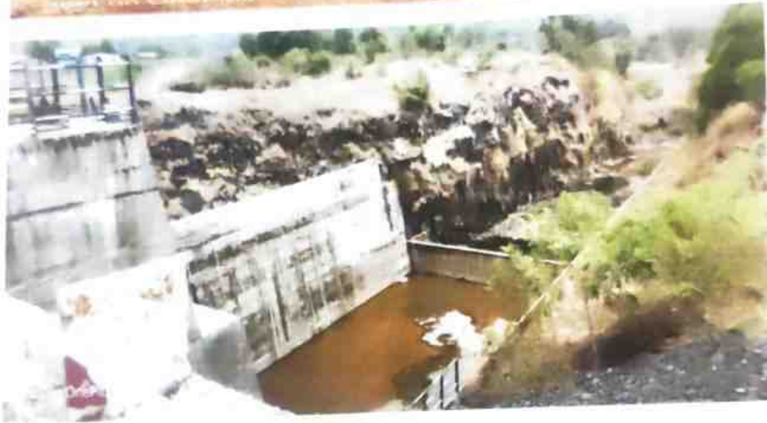
Photo :Ogee Spillway at Gunjawani dam
