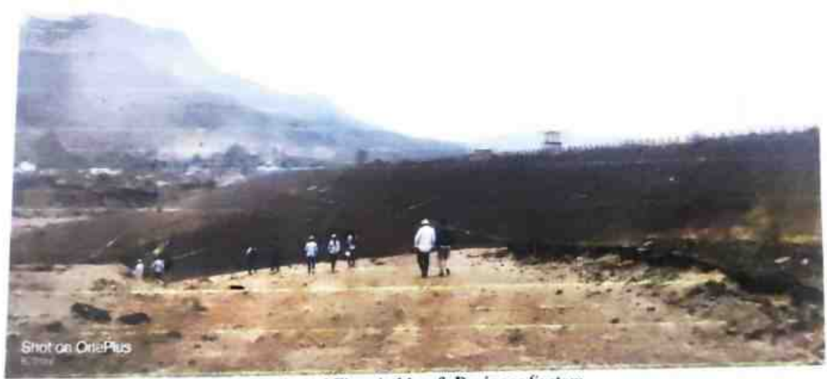
Photo . Needle and Flat pitching & Drainage System
