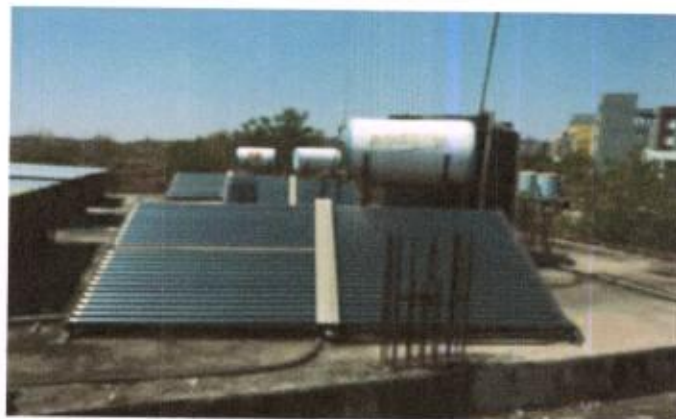
Photograph of Solar Thermal Water Heating System at Hostel block:
