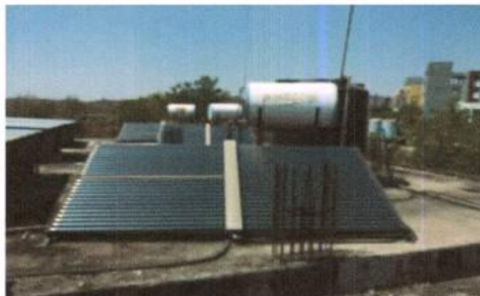
4.3 Photograph of Solar Thermal Water Heating System at Hostel block:
