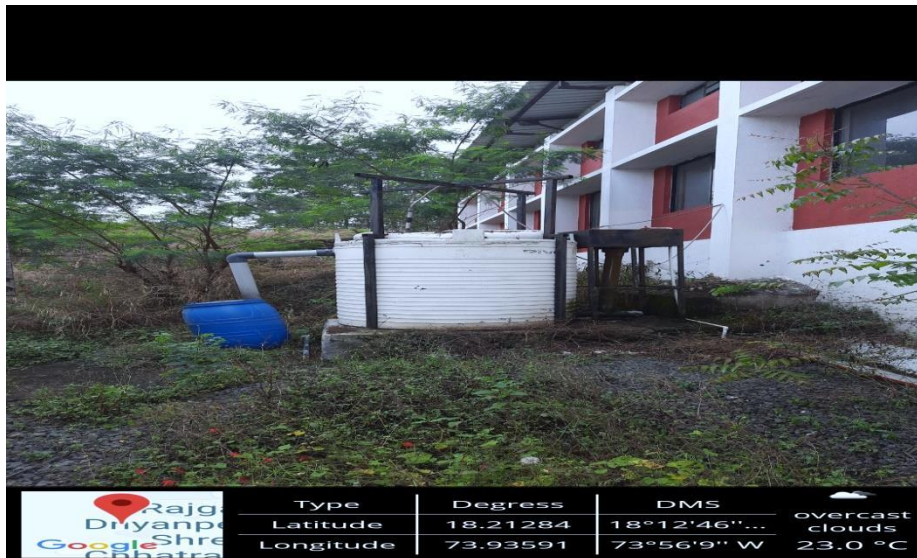
Bio Gas Plant
